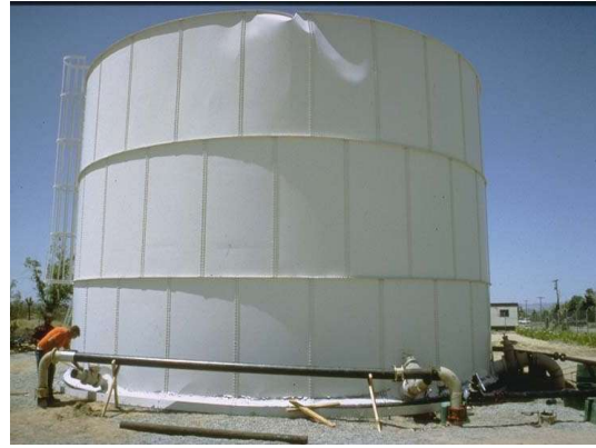
Figure 2. Shell buckling [22]
