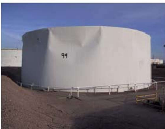
Figure 1. Roof buckling [21]
