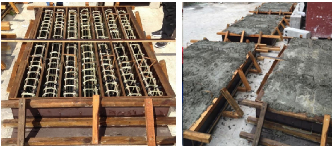
Fig. 3 Production of the beams
