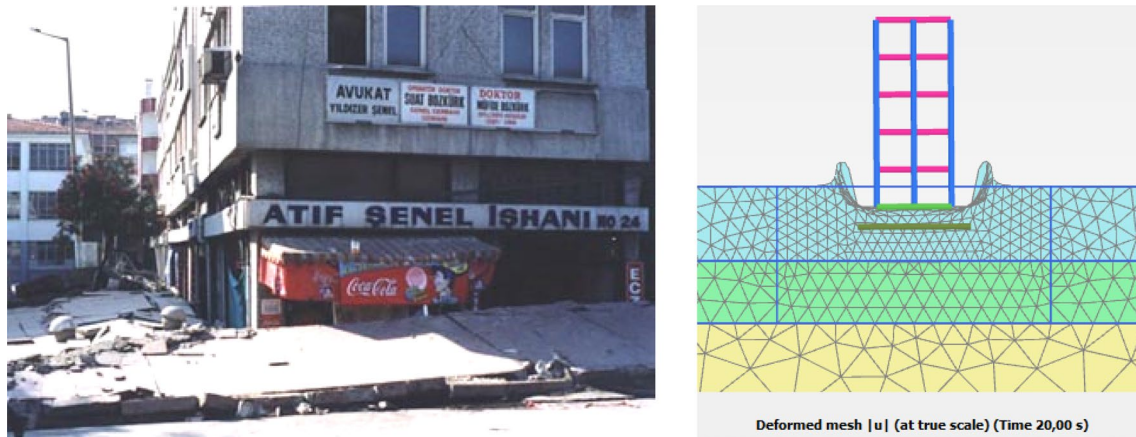
Fig. 8 The response of the actual building in Marmara Earthquake and the FEA Model
